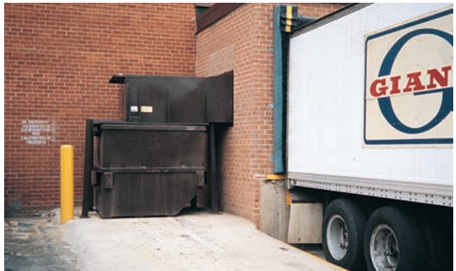
Installed at a supermarket, this side feed VIP is equipped with an optional "thru-the-wall" security chute enabling the unit to be fed from inside the building. The security chute controls employee pilferage by eliminating the temptation to put merchandise into a box, stash the box in a trash container and return at night to retrieve the merchandise. The refuse is totally enclosed with no access to scavengers.
